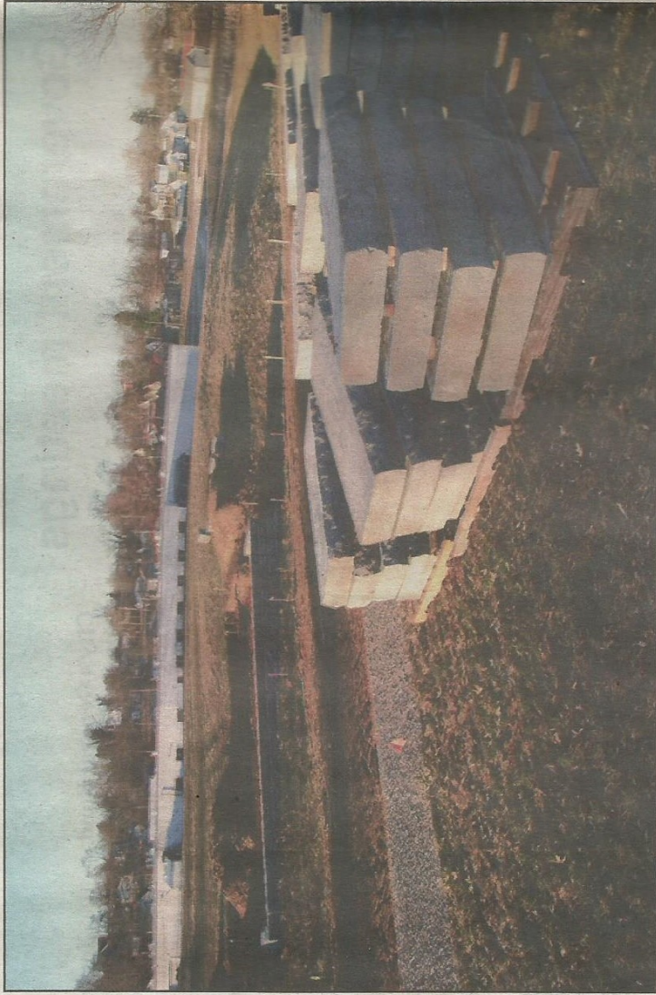
The area where the amphitheater "stage" will be located is seen as a rectangular structure at mid left. Directly across from the stage area will be ascending levels five and a half feet to eight feet wide with the stones at right providing seating at the rear of each level. —Staff Photos by Barbara King
